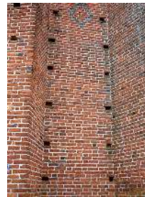
restrained console scaffolding
