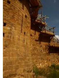
restrained console scaffolding
